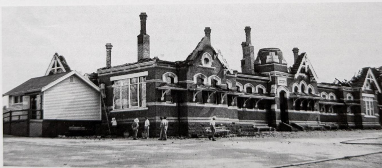
Fig. 20 'Camperdown State School No. 114 : Destroyed by Fire in February 1965 [CDHS Collection]
