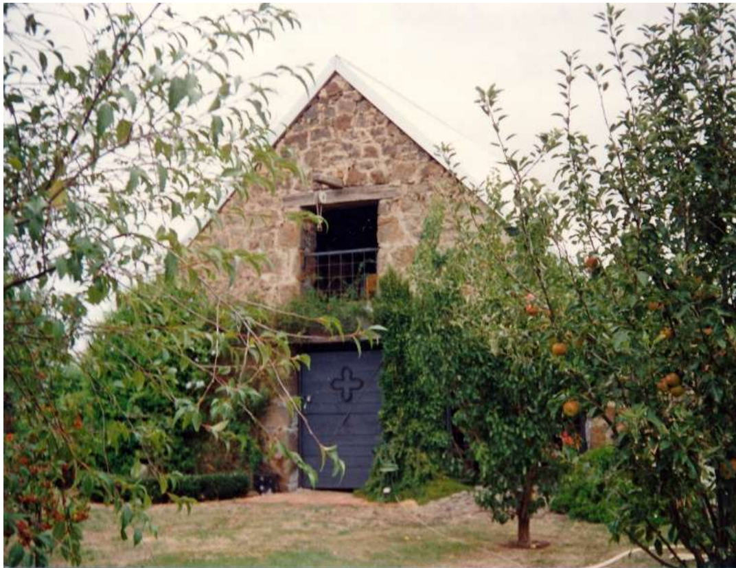
Former 'Stony Rises Hotel Stables', half way between Colac and Camperdown
