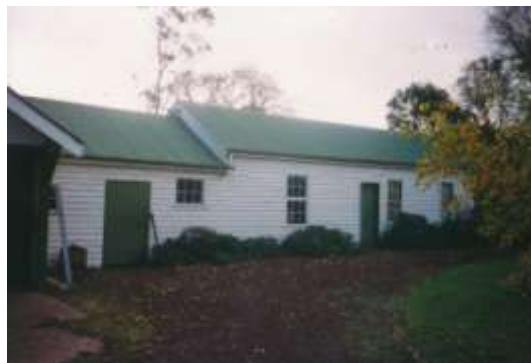
"Wuurong" - timber addition to the building c.1984
